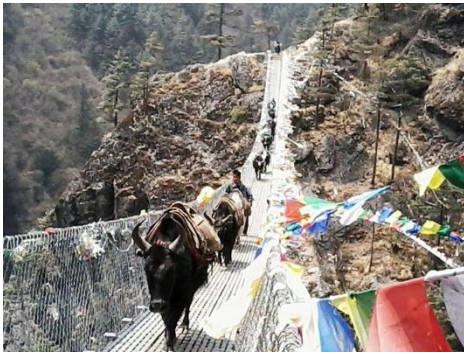
Crossing over suspension bridge
